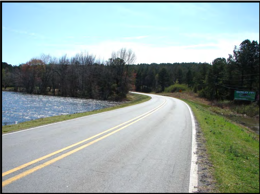
Figure 11 - View to the south from the northern terminus of the project (Highway 25 at Beaver Fork Lake)
