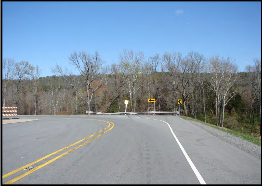
Figure 10 - View to the north of Blaney Hill from the southern terminus of the project (I-40/Hwy. 64 Spur interchange)
